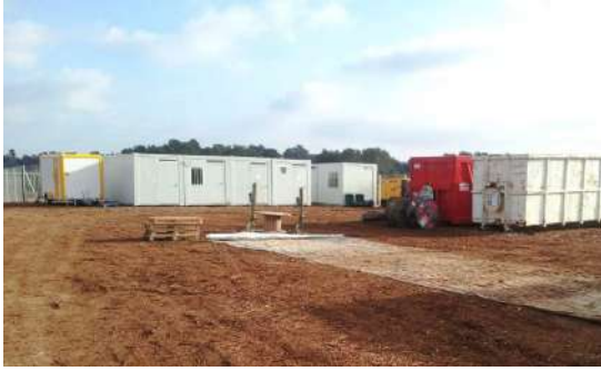
Installation de la base vie
